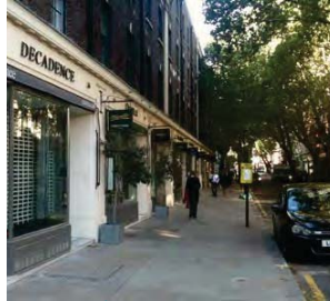
Shopfronts in one storey retail plinth
