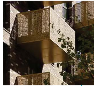
Metal projecting balconies
