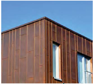
Copper clad top floors with setbacks
