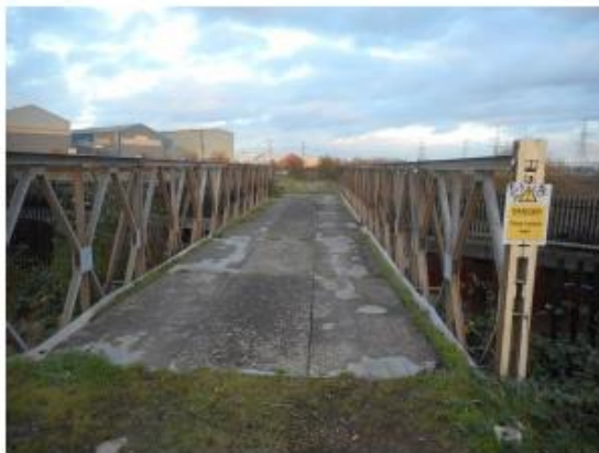
Pymme's Brook Bridge
