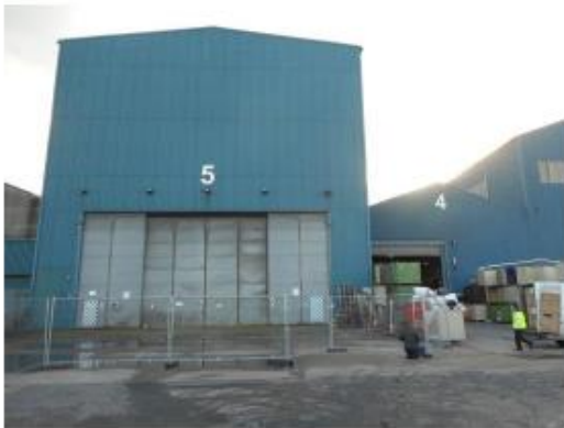
Front Elevation to Units 4 and 5
