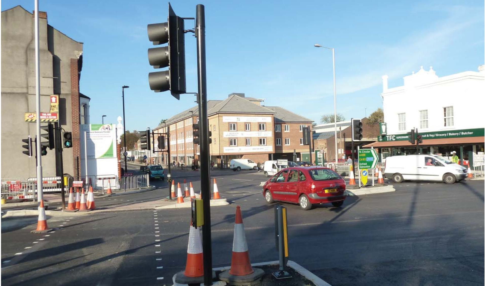
Green Lanes/A406 junction
