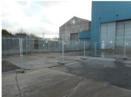
Forecourts to the front of Units 5 and 6
