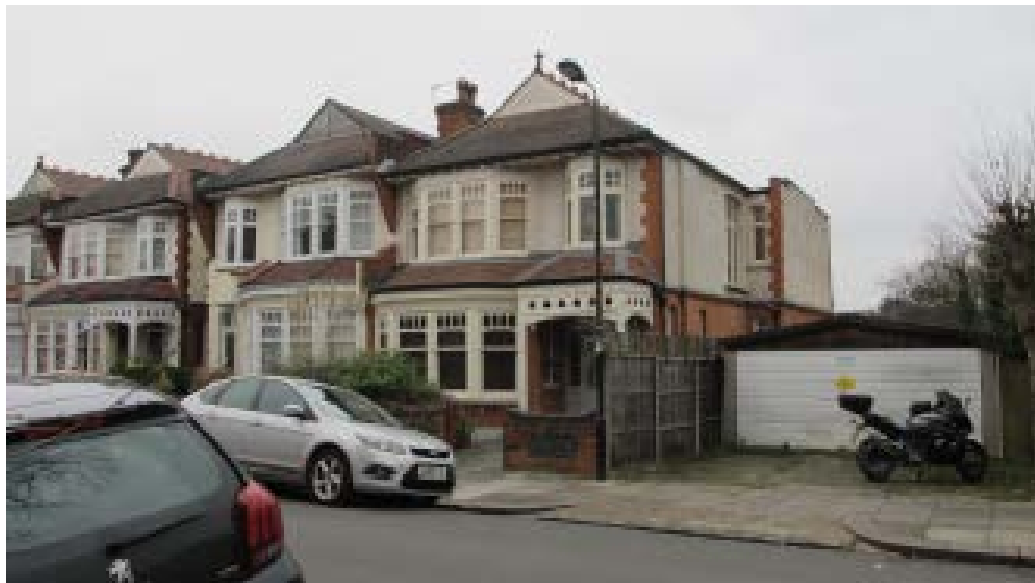
Photo 2 - Burford Gardens Elevation showing Existing Crossover and detached garage to be retained and No. 2 Burford Gardens to the left side.
