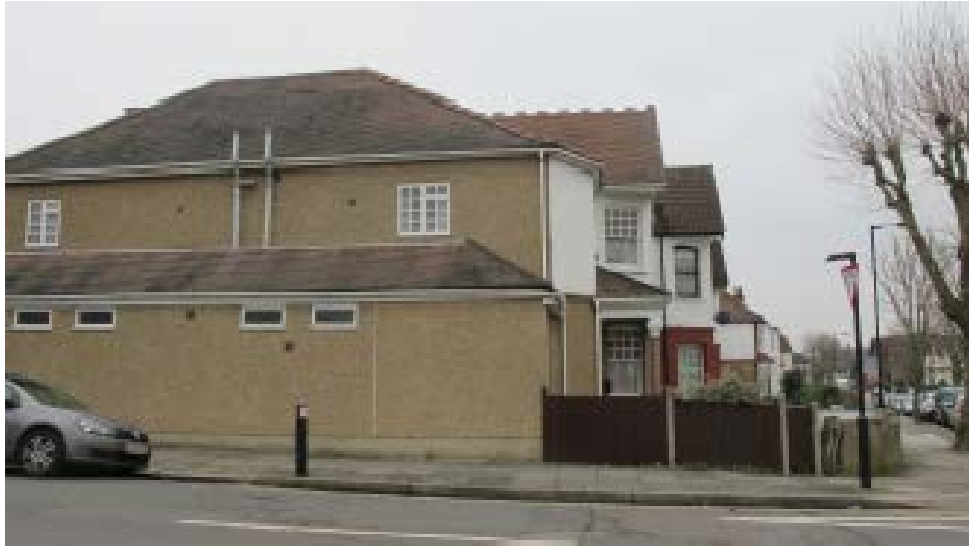
Photo 3 Flank Elevation – Burford Gardens side
