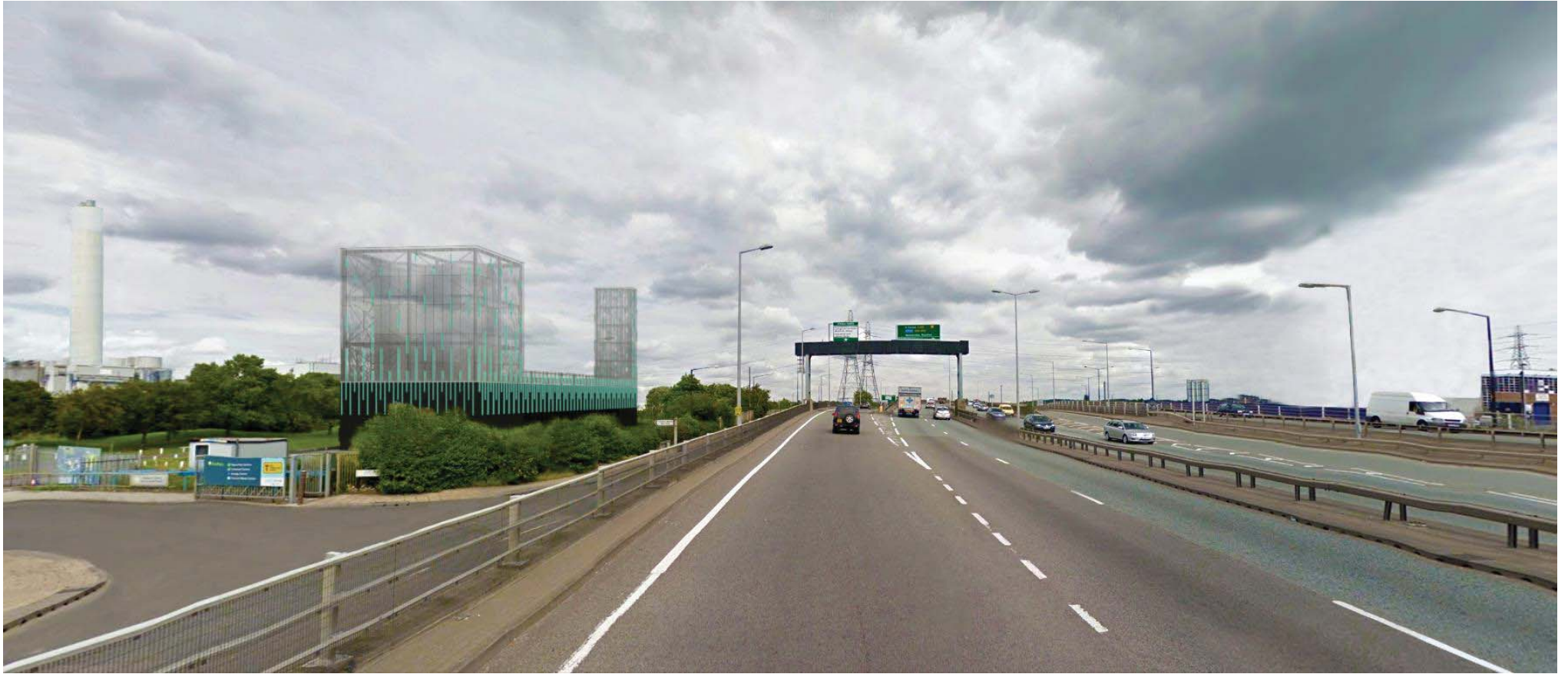
View from North Circular - Eastward
