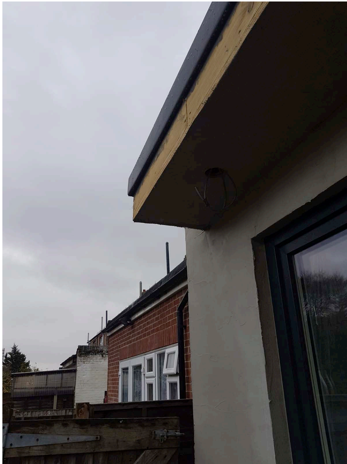
1 Canopy at east side - work in progress
