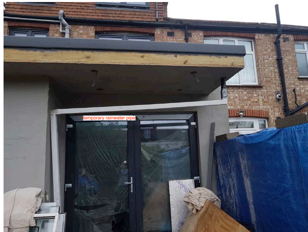
2 Canopy viewed from garden - work in progress
