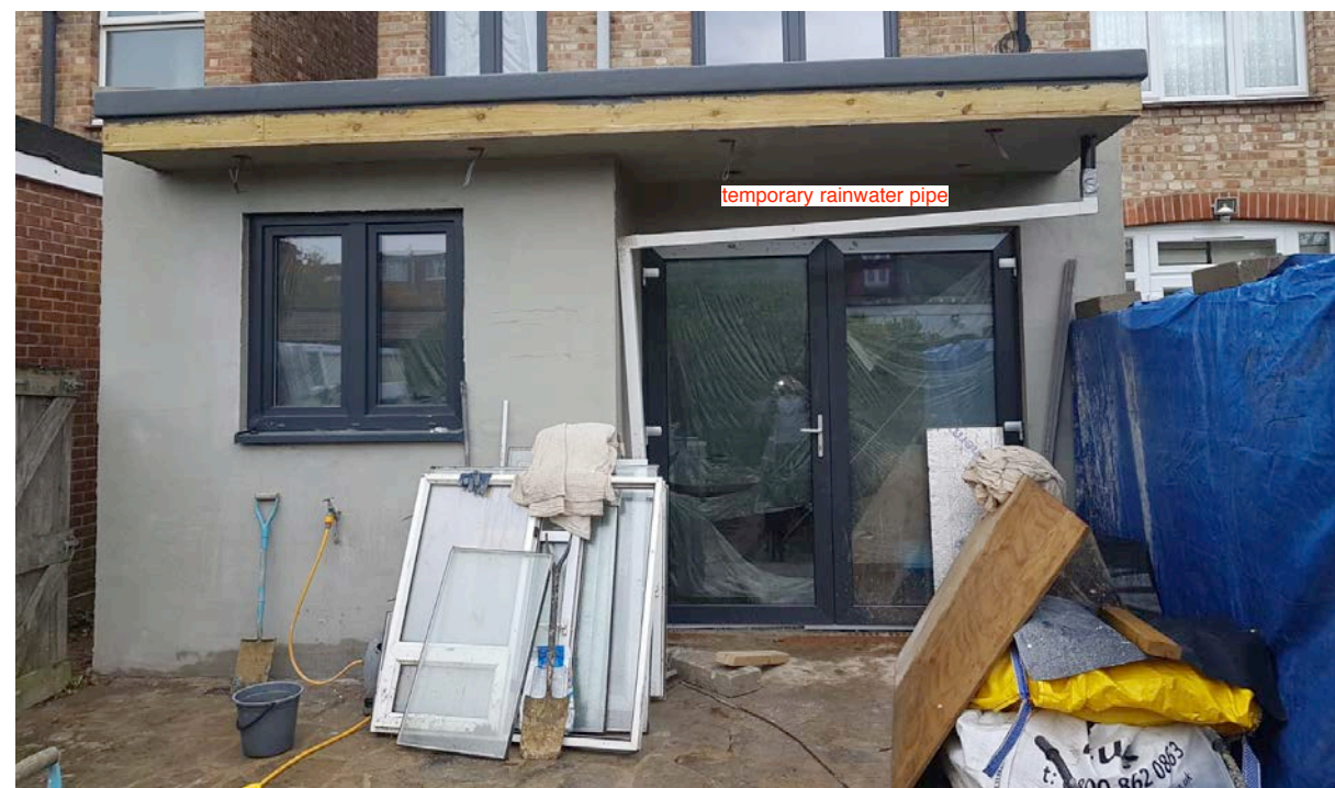
3 Canopy viewed from garden - work in progress
