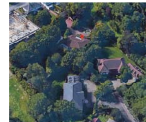
NOTE: LARGE AMOUNT OF TREES BETWEEN NO.9/10 ALDERWOOD MEWS AND APPLICATION SITE TO BE RETAINED
