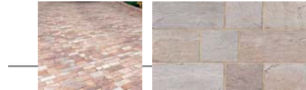
Example of cobble sets drive laid in random stretcher bond Example of buff and brown paving mix
