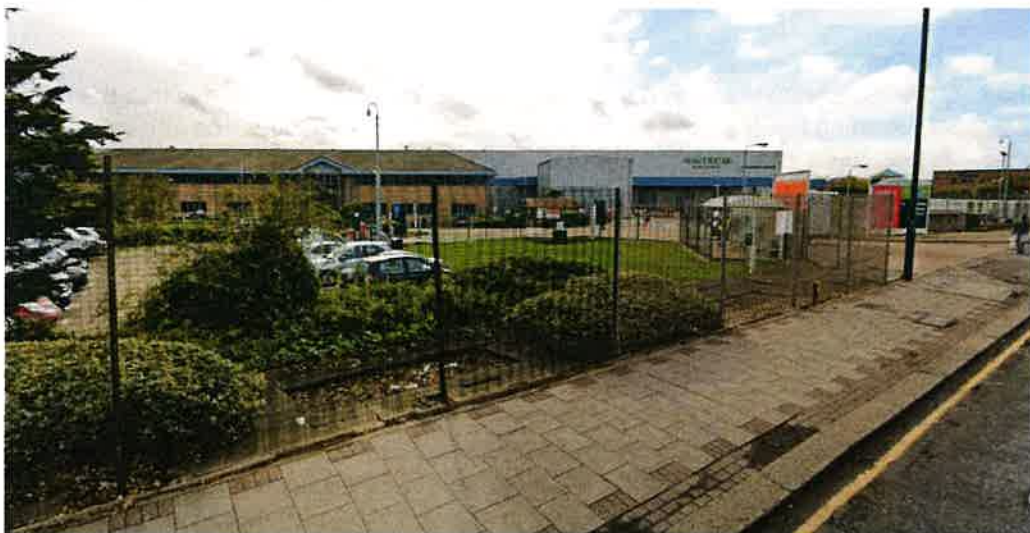
Figure 4: Existing poor streetscape along Southbury Road
